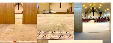
Would be good during install to properly mark the cabling for the loop system. Otherwise it is 'just' a cable under the carpet/ground. Picture taken from contacta.
